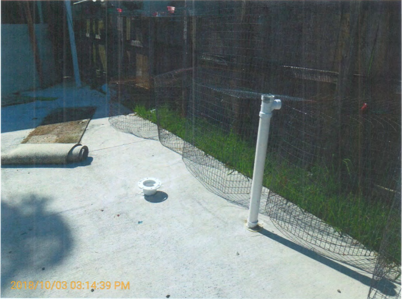
Plumbing piping in rear slab to be removed
