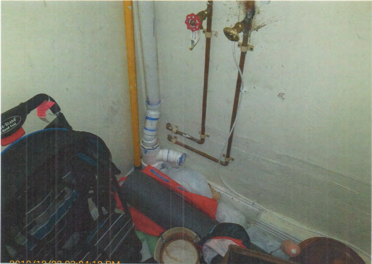
Illegal efficiency in garage area to legalize or demolish
