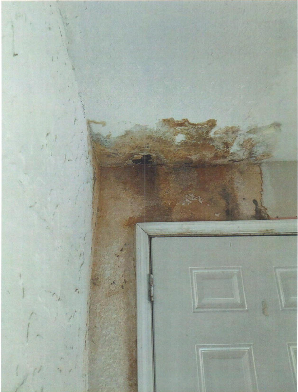
Water damage (rear addition)
