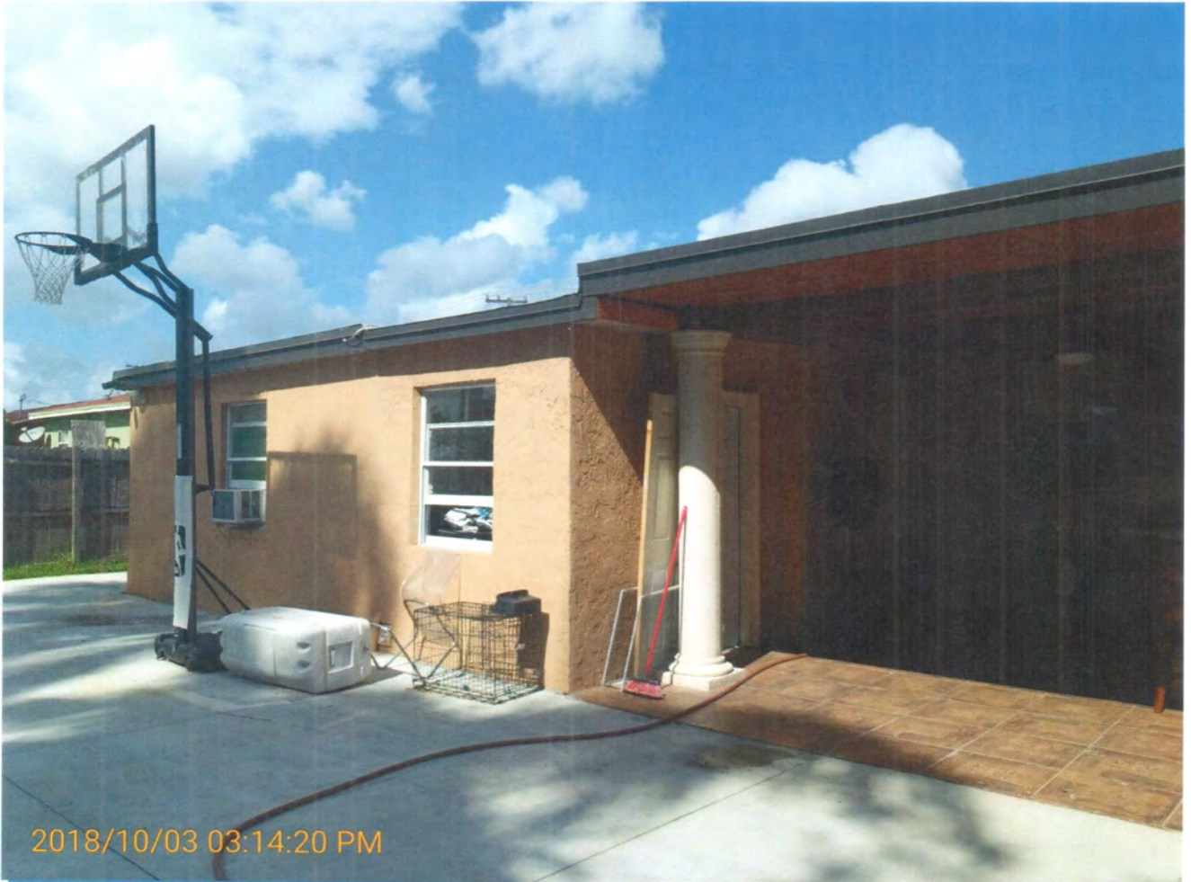
Illegal rear terrace and additions (3) to legalize or demolish
